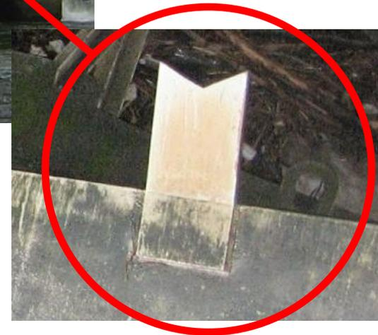
Division of the stream with the help of "swallow tails" ensures the inflow of air under the stream and prevents aspiration and accompanying cavitation of the structure.
