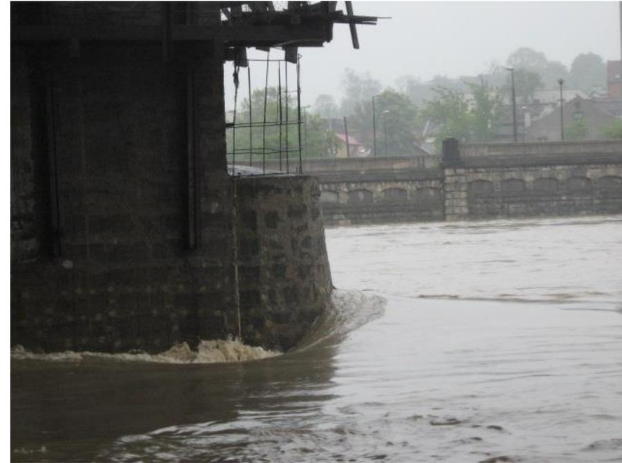
Elevated watertable and acceleration of flow at the pillars of the Grunwaldzki and railway bridge in Kraków (increased velocity magnitude at the pier walls cause increased bottom erosion in these places)
