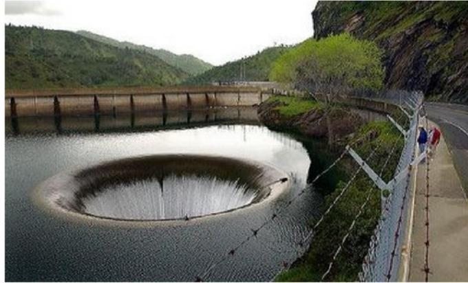
Shaft weir in Monticello (California)
