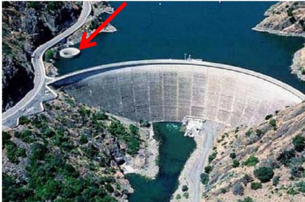
Inlet and outlet of the shaft weir Monticello
