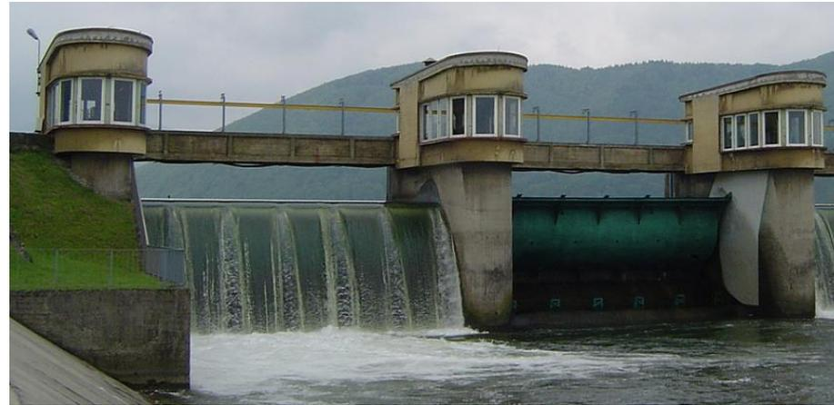
Hydraulic structures used for discharging flow from reservoir into downstream part of river channel.
