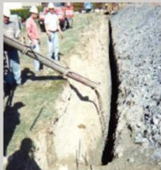
Unsupported trench (20 ft, 6 m)
