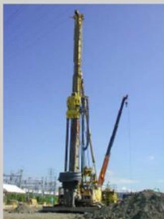
Soil mixing (40 ft, 12 m)
