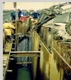
Cofferdam (30 ft, 9 m)
