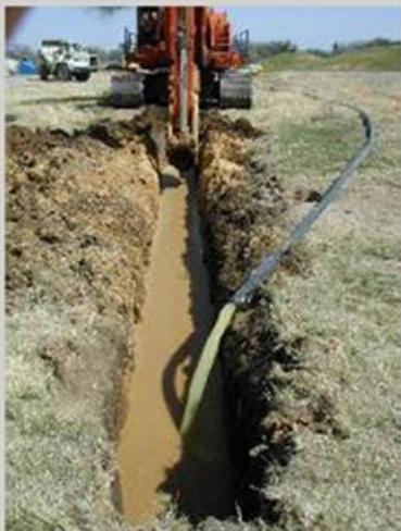
Trench supported with liquid polymer (70 ft, 21 m)
