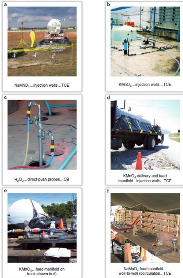
Figure 1.11. Photographs illustrating some of the conditions and infrastructure at sites where ISCO has been deployed for groundwater remediation. Image captions give oxidant used, delivery method, and target contaminants. Note: CB - chlorobenzene, MGP - manufactured gas plant.
